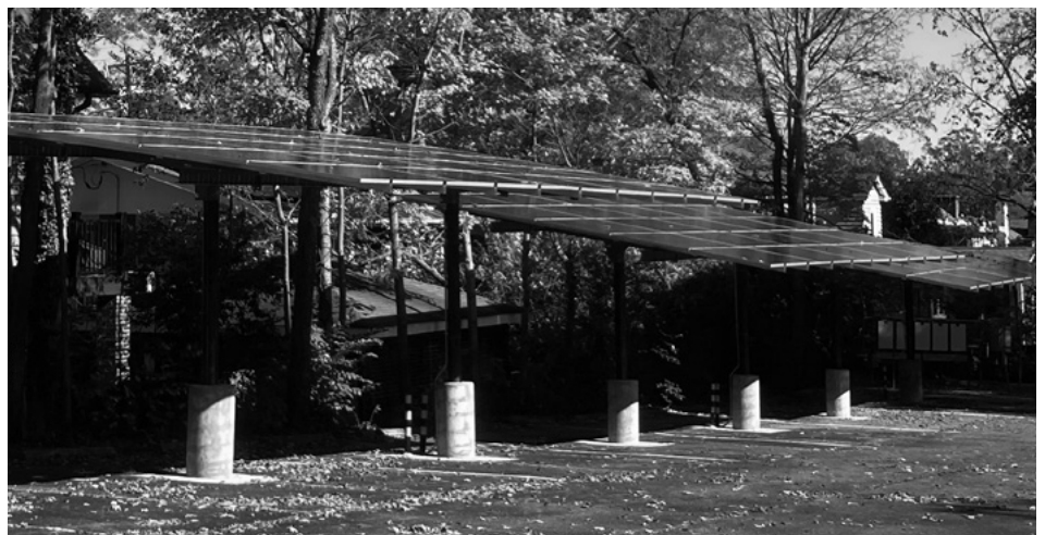
Solar carport at Watts Street Baptist Church
